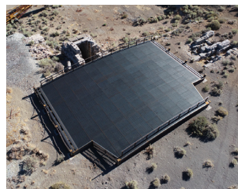
Completed cupola over Forman Shaft
