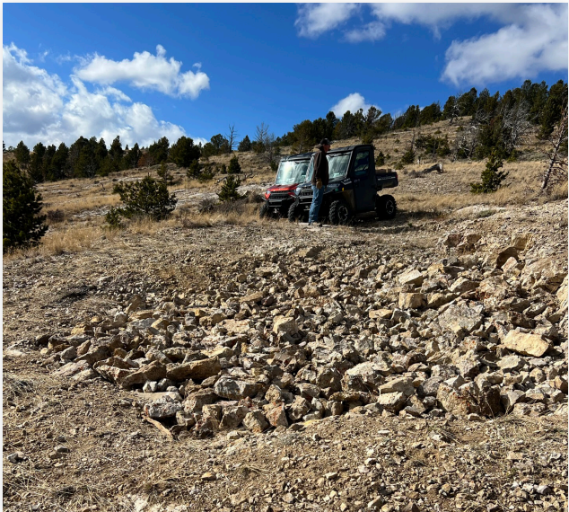
BLM-State partnership closure. Bald Mountain Uranium Shaft Closure. Carbon County, Wyoming
