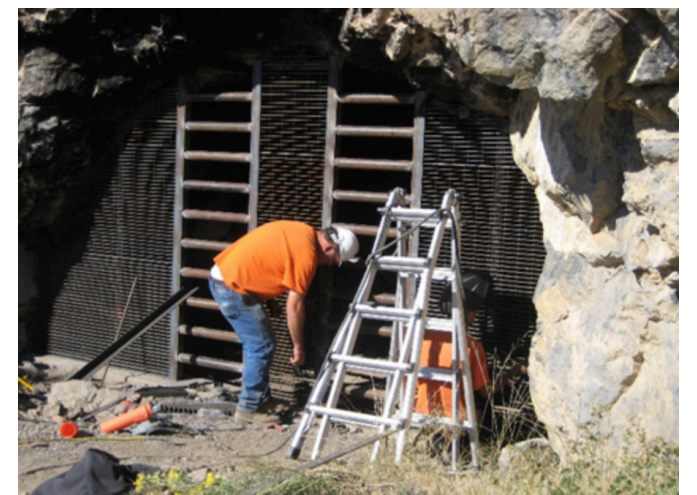
Bat Accessible Closure, Fremont County, CO.
