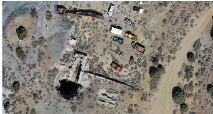
Over head image of Forman Shaft before closure. Note the size of the shaft compared to the abandoned equipment on the site.
