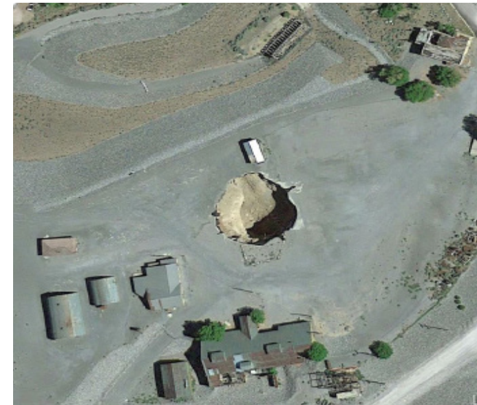
Aerial image of the Chief No. 1 shaft subsidence. The subsidence feature in the center is approximately 100 ft. diameter.
