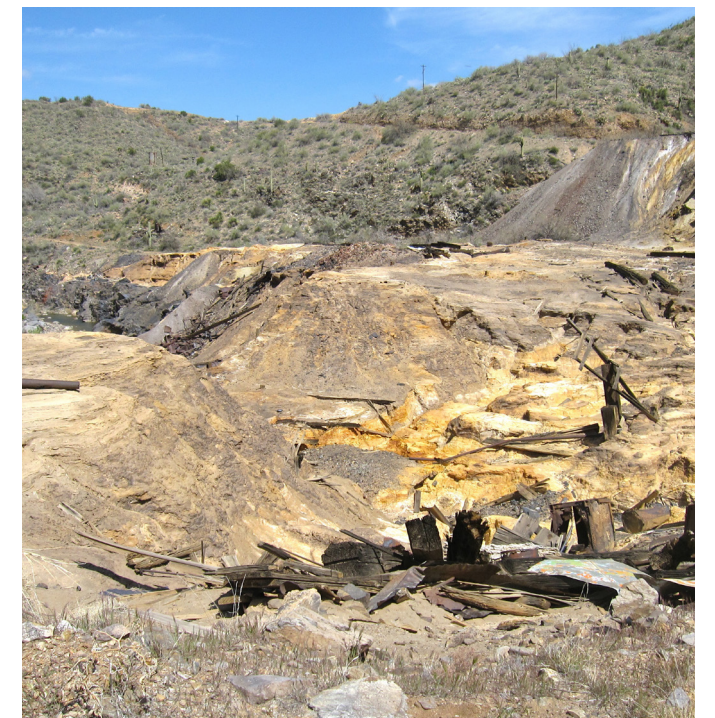
Safety and environmental hazards at Hillside Mine in Yavapai County, Arizona
