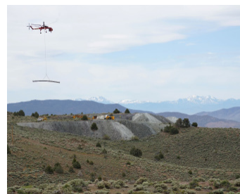
Skycrane flying one of the 80' long support beams
