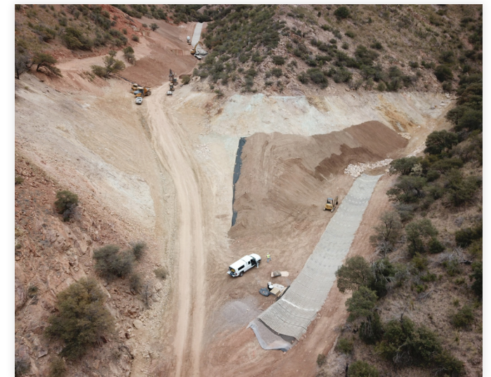
Reclamation at 3R Mine in Santa Cruz County, Arizona
