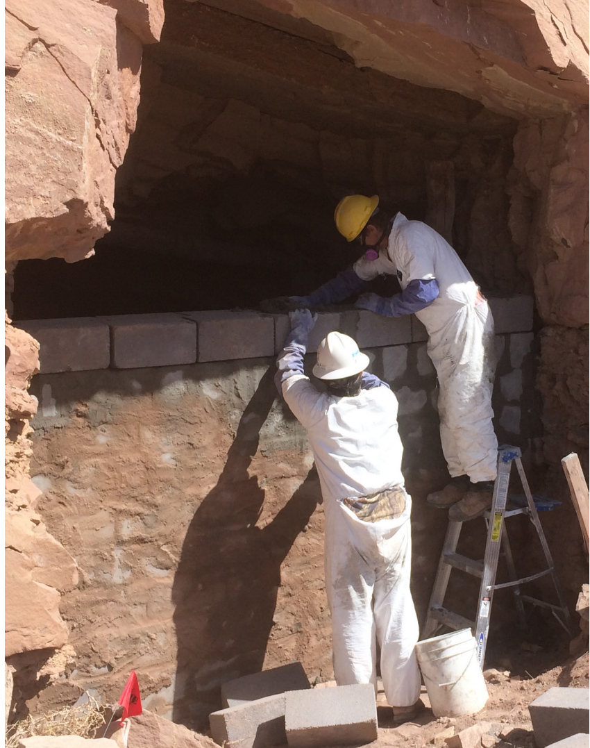
Workers constructing a block wall closure at an abandoned uranium mine adit wearing protective clothing and respirators. San Juan County, Utah
