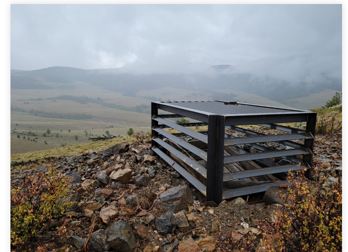
Bat Cupola closure over mine shaft, Carbon County, Wyoming
