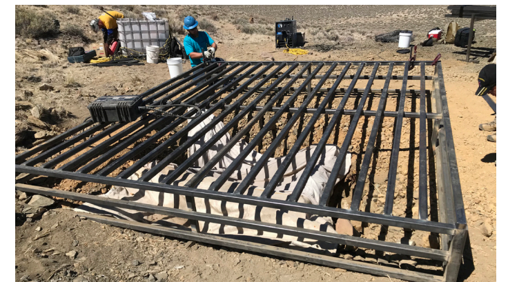
Finishing a bat cupola over a shaft with tarps protecting the timber below
